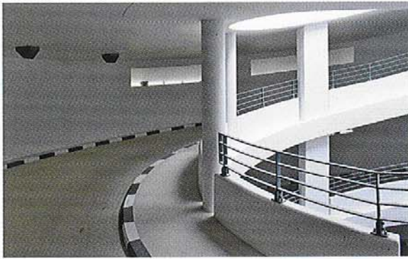
Image 109: EAR 05-compliant spiral ramp with all the required safety features ( Alter Steinweg, Münster )
