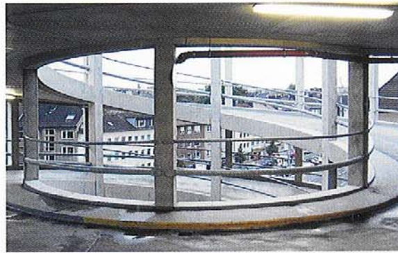
Image 110: Almost fully rule-compliant, highly transparent spiral ramp. This ramp, however, fails to provide safety kerbs on its outer side
