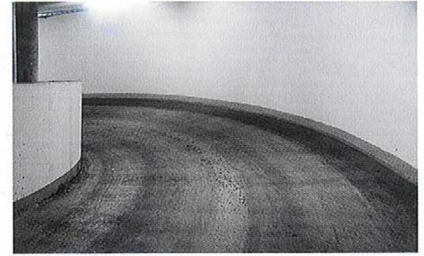
Image 111: Spiral ramp with an only 3.50 metre wide driving lane without safety kerbs and guidance aids
